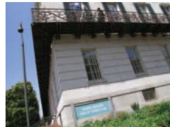
An exterior surveillance camera mounted on a post contoured to blend with nearby streetlights eliminates the need to penetrate or visually alter the facade. The camera's globe housing and post have been patinated to read as a single assembly.
