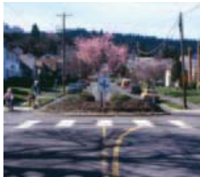
Bicycle boulevards may include traffic calming devices like traffic circles. Courtesy Portland Office of Transportation
