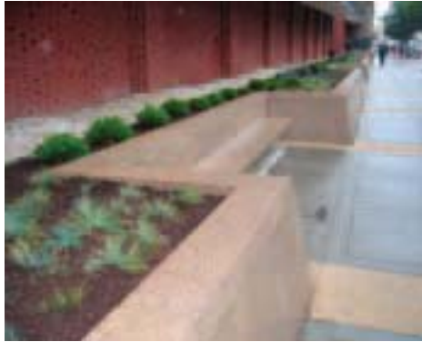
The perimeter around the New Executive Office Building in Washington, D.C., includes transparent security in the form of street furniture and landscaping.
