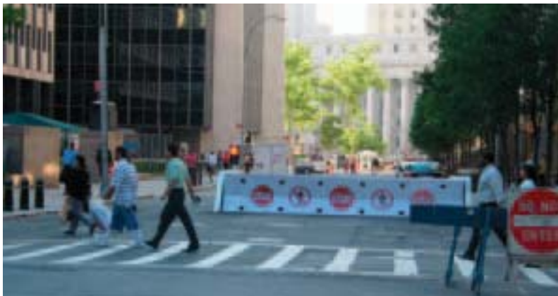
Concrete barrier limits vehicles at Federal Plaza, Duane Street, Lower Manhattan, N.Y.
