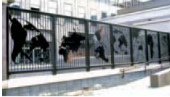
Integrating public art with perimeter security. “Pangea Fence,” at Townsend Harris High School, Flushing, Queens, New York.
